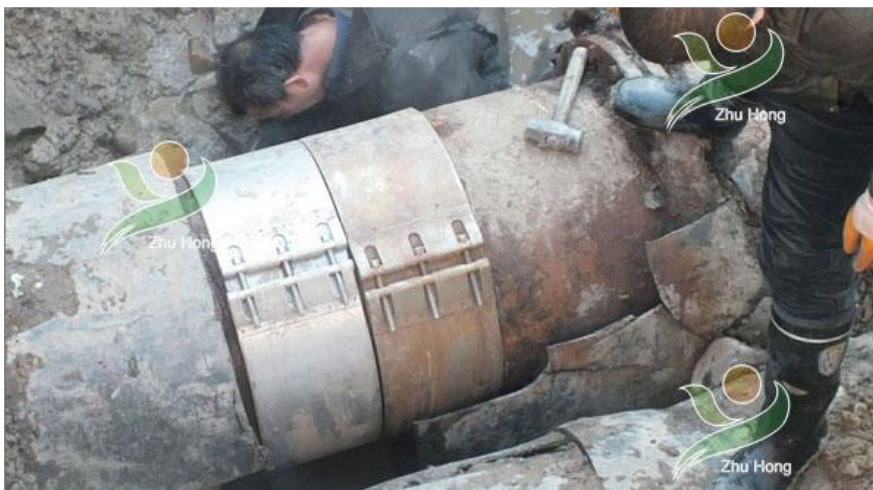
Figure 2. Pipe repair using pipe clamps [7].
